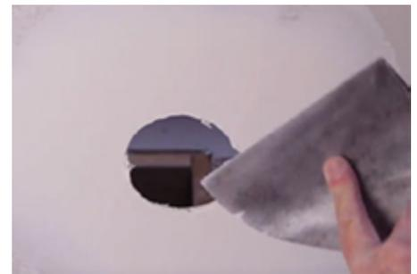
Step 3. Then apply a slightly wider second coat of plaster and flatten it out to make the repair less visible. Repeat the process with extra layer of finishing compound.
