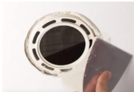
Step 2. Apply the first coat of plaster. Hold the plate ensuring it doesn't move. Remove any excess product from the inner ring and scrape the surface until it's flush with the ceiling.
