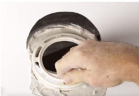
Step 1. Apply sufficient plaster to the wings to ensure it holds securely in the ceiling, and place the kit to the ceiling cavity and pull down onto the ceiling surface.
